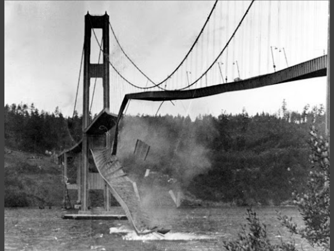
Tacoma Narrows suspension bridge Massive but structurally flawed and failed catastrophically
